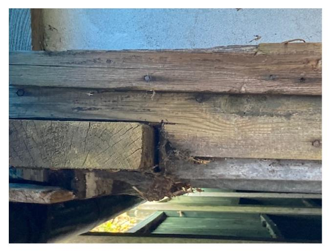
This shows from the outside, the corner where the toilet is, with tin sheets running along next to **short**. Please note it is a wooden shed with galvanised tin sheet cladding to outside. As you see the tin sheets stop short of the plastic roof. The gap
